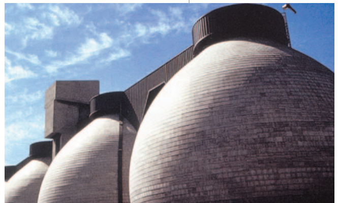
Egg-shaped Digestors
